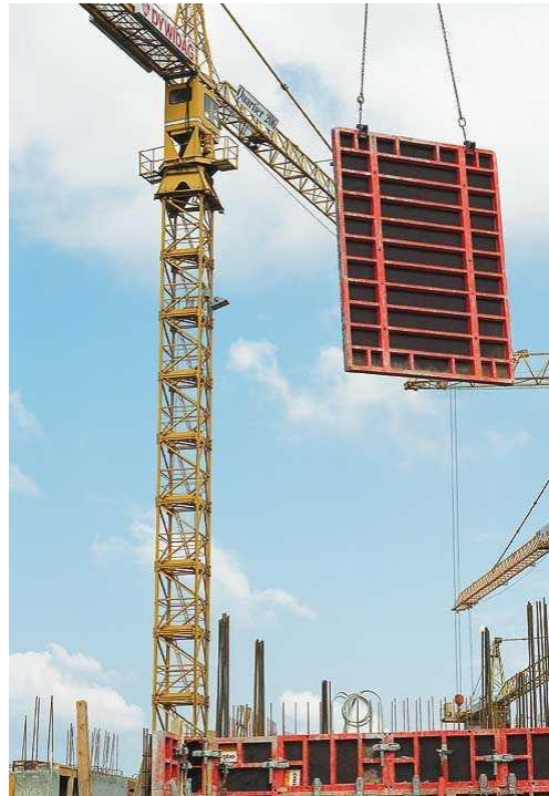
Figure 2.21 Illustrating the use of wood-based panels in formwork.
