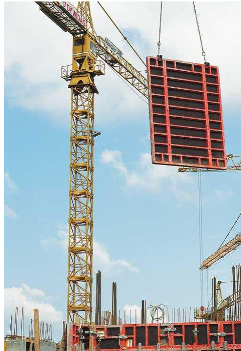
Figure 2.21 Illustrating the use of wood-based panels in formwork.
