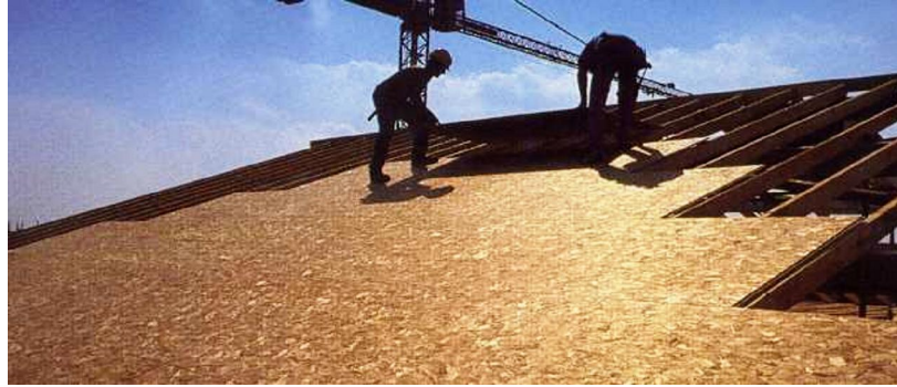
Figure 2.12 The use of OSB for sarking
